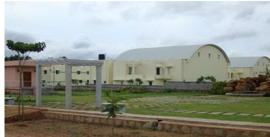
Doddaballapur Integrated Textile Park, Karnataka
